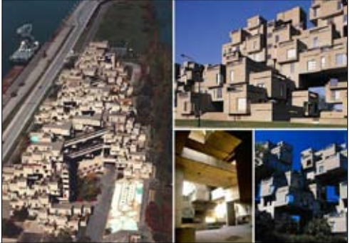
This is Habitat at Expo '67 in Montreal designed by Moshe Safdie. Basic units connect together in an irregular pattern. This creates usable negative, exterior wall, and roof space.
